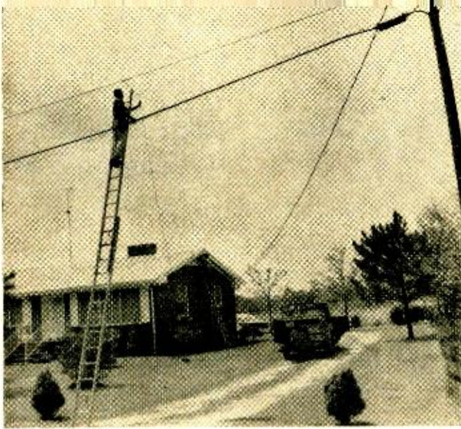
Lineman installing tap-off connecting subscriber's home to cable.
