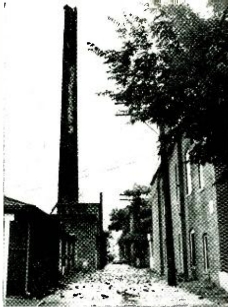
Chimney shows severe damage which was caused by a lightning stroke.
