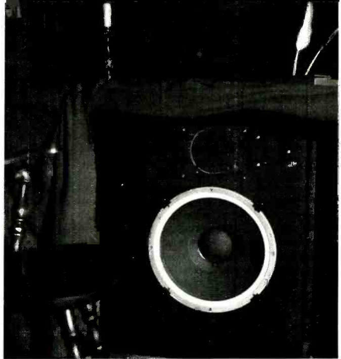
One of modified speaker systems located under ten tables in the Assembly Hall. Theater drivers are used for the middle and upper frequency ranges along with woofer for desired bass.
