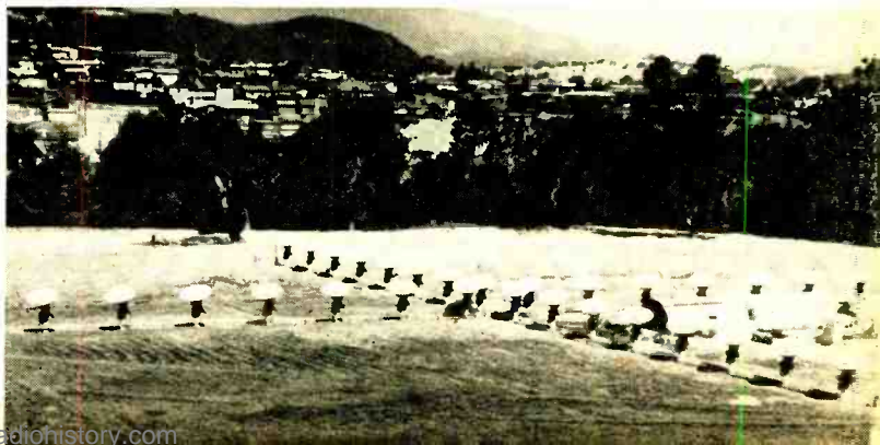
Fig. 7. Stanford University's 375-ft. pencil-beam cross interferometer consists of 32 interconnected 10-ft. reflector dishes.
