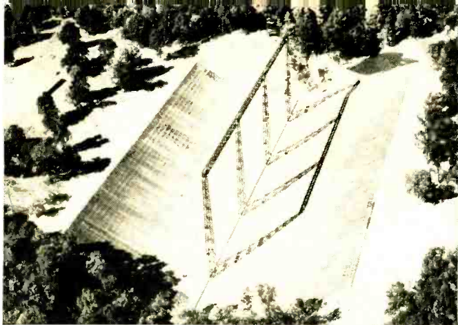
Fig. 4. The University of Illinois parabolic cylinder antenna. This particular radio telescope uses electronic beam scanning.
