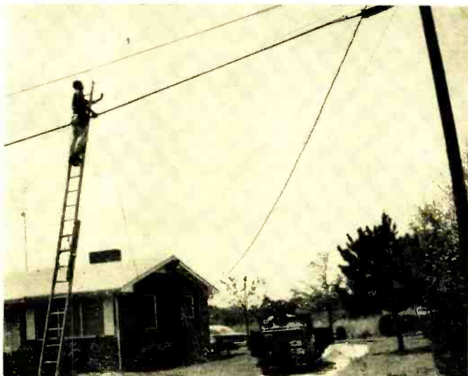
Service team installs droplines from the main feeder cable.
