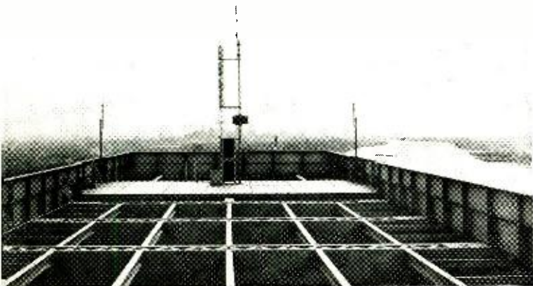
Fig. 3. Adler translator installation at east end of G. Washington Bridge faces famed New York skyline, in background.
