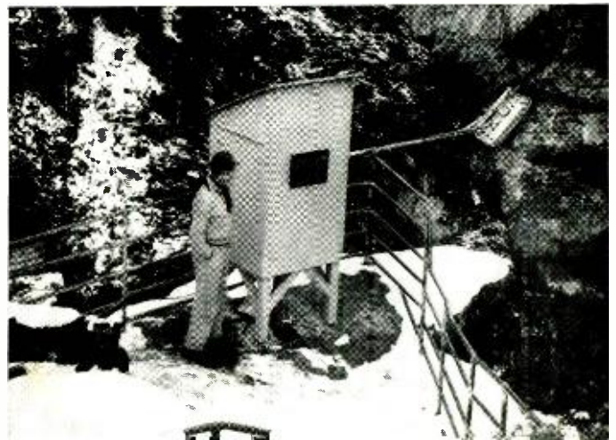
Fig. 7. This translator's u.h.f. antenna (mounted on arm) shoots into deep valley at Yosemite National Park, bringing TV to a signal-blocked community of forest-ranger families.
