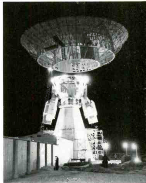
Step 1. The nine-ton "Advent" antenna reflector is shown resting on the ground prior to its being hoisted atop its three-story pedestal shown at left in this photo. Step 2. The 60-foot reflector is being hoisted into place by means of 200-foot heavy-duty construction-type cranes. Step 3. The cranes have just been removed from the giant reflector which is resting securely in place on pedestal.
