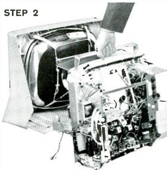
Just two more screws remove the entire chassis! If it ever becomes necessary to pull the chassis, simply remove two more screws and lift it out. The duallette carrying handle becomes a carrying handle for the chassis!
