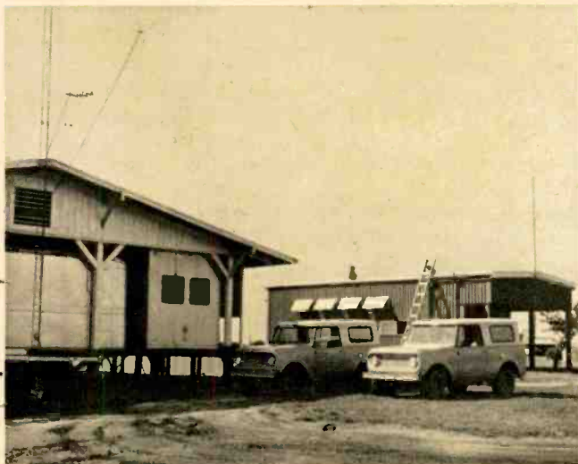
Transmitter building (left) is made up of trucks under roof. Power station is in the background.
