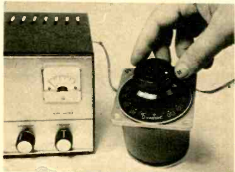
Variac (right) controls voltage of incoming house current in test of effect on RF output power of CB rig (What Price Power?, opposite column).
