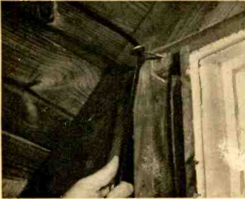
TV standoff insulators support antenna at each end. Use standoffs between center board and the end supports wherever antenna arms might sag.
