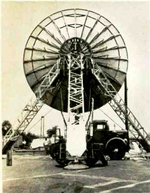
Antennas for scatter systems are among the most photogenic going. The back-to-back pair above, located in the Aleutians, relay messages in opposite directions to points hundreds of miles apart. Designed for military use, the mobile antenna on left can be erected most anywhere. It's strong enough to withstand 120-mph winds, once it's anchored.
