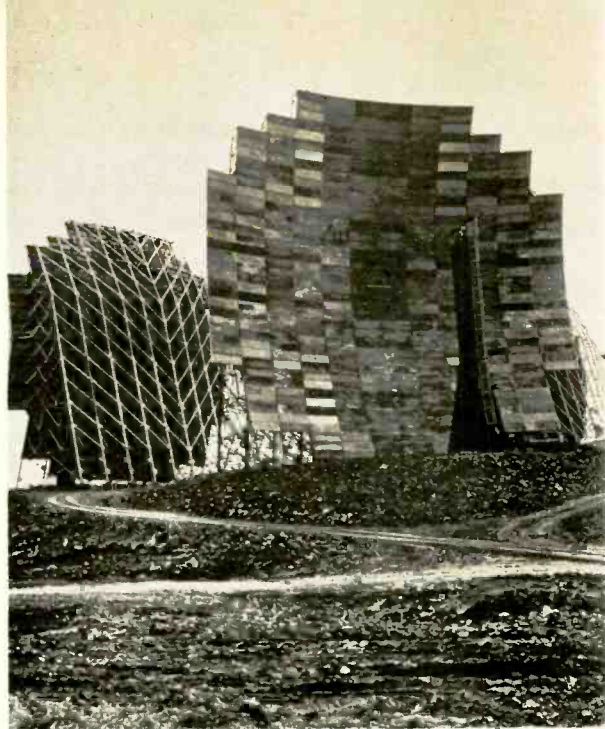
Antennas for scatter systems are among the most photogenic going. The back-to-back pair above, located in the Aleutians, relay messages in opposite directions to points hundreds of miles apart. Designed for military use, the mobile antenna on left can be erected most anywhere. It's strong enough to withstand 120-mph winds, once it's anchored.
