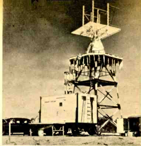
One of four "command" tracking stations in the 18-station net is at Muchea, Western Australia.
