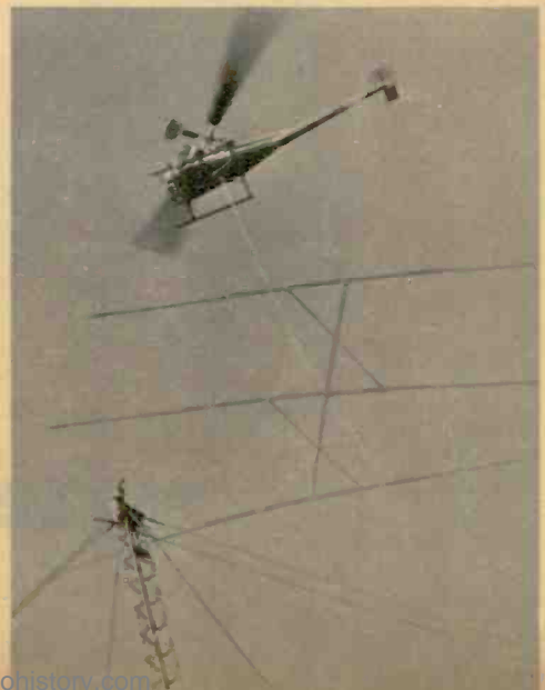
Hams, attention! Why labor to put up a beam? Hiller Co. helicopters put up two beams at Stanford U. Radioscience Lab in 16 minutes.
