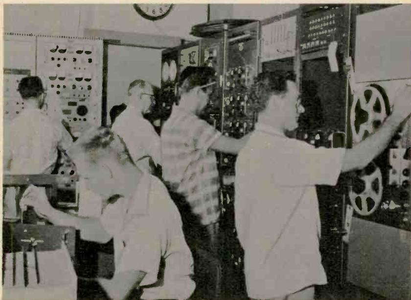
Complex telemetry racks for rocket firing, guidance and data gathering get serviced and modified almost constantly to avoid hitches when the chips are down.
