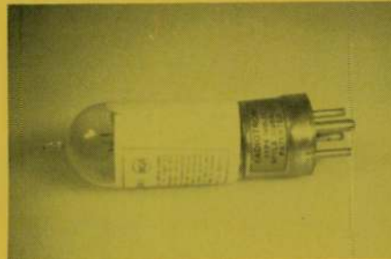
Fig. 1 The WD-11 "peanut" tube was 4-¼ inches in length.
