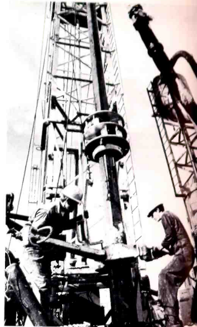
Westinghouse Electric Corporation Drilling Rigs for Rescue
