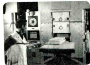
Base materials are fired to form the phosphors
