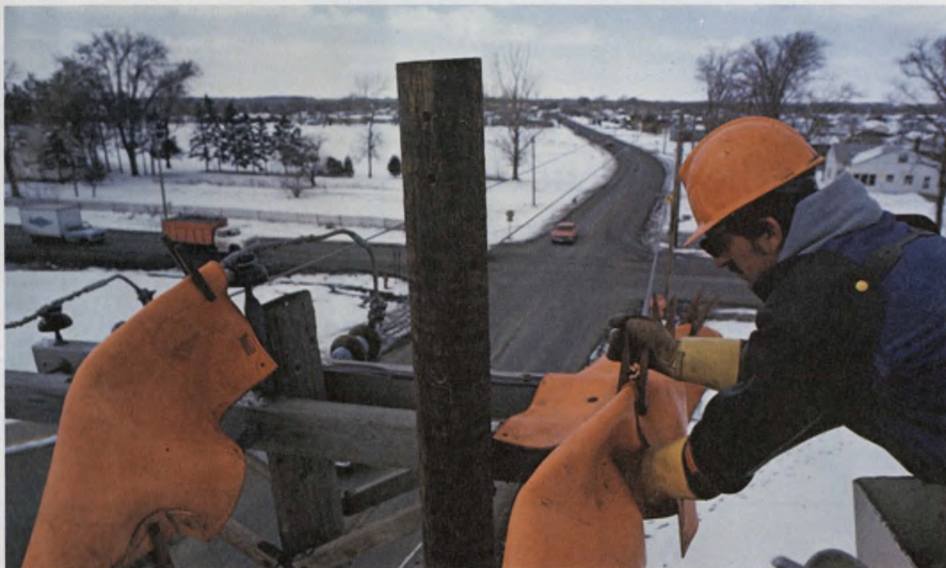
To increase the power available to customers in Fridley, Minn., a Northern States Power Co. construction crew is converting a single-phase 13,800-volt line to three-phase service.
