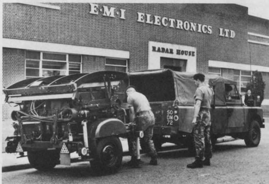
Highly mobile mortar locating radar developed for the British Army is mounted on a two-wheeled trailer.
