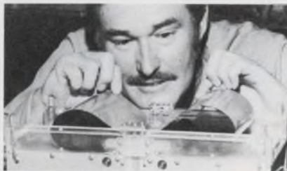
Project engineer Charles Davis watches piezoelectric material advance film.
