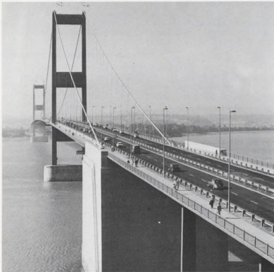
The Severn Bridge, connecting England and Wales, uses a computer-based toll collection system that also issues ice and fog warnings.
