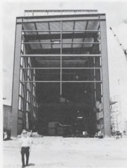
The deep-sea simulator to accommodate both man and submersible will go into this three-story structure at the naval base in Panama City, Fla.
