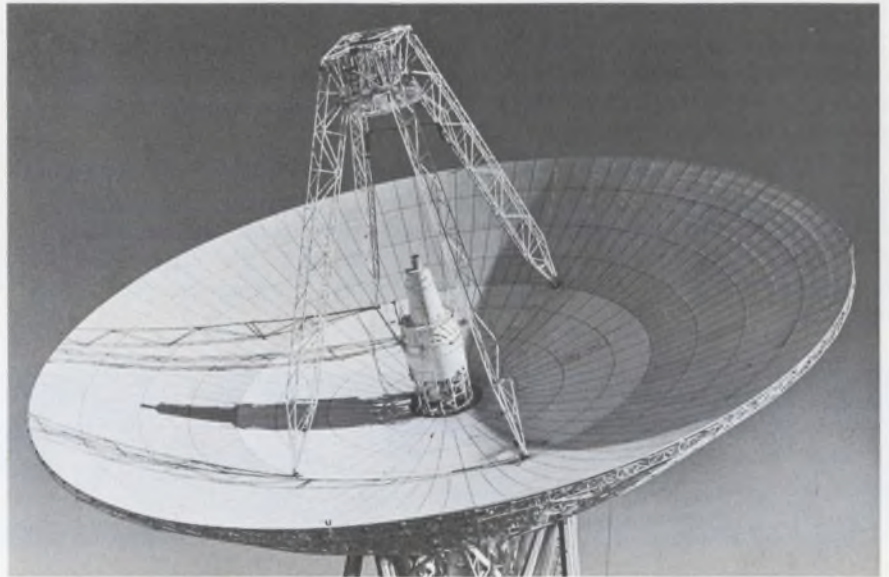
Transmission of data from Mars at 16,000 bits per second became feasible when a 210-foot antenna went into operation. The result: best photos yet taken of the planet. p. 25.
