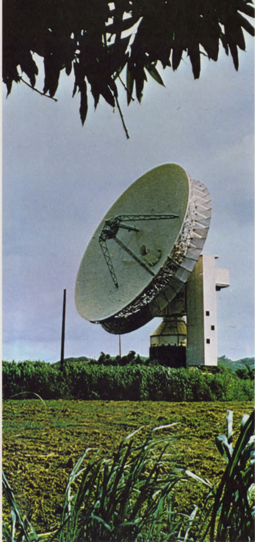
Looming up out of a field of cane at Cayey, Puerto Rico is this 85-foot earth station antenna. The station links the island with the U. S. mainland, Latin America, Europe and other Atlantic Basin points equipped with earth stations.
