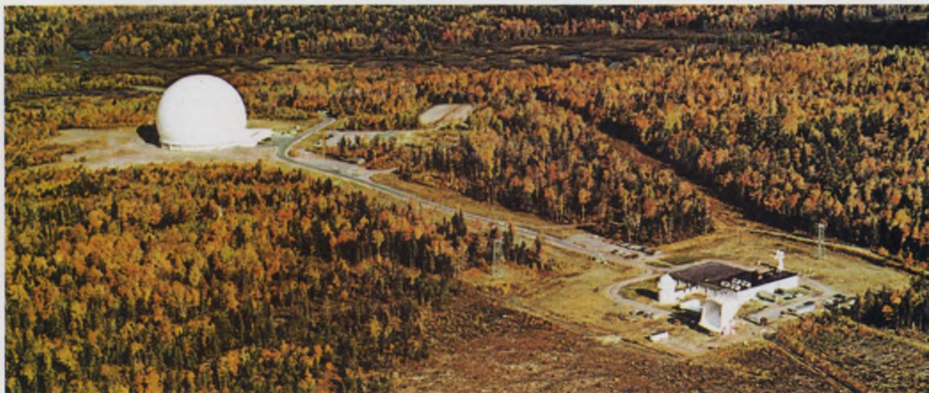
A huge 380-ton horn antenna is housed in this radome nestled in the autumn foliage near Andover, Maine. Originally built by Bell Telephone Laboratories for exper-
