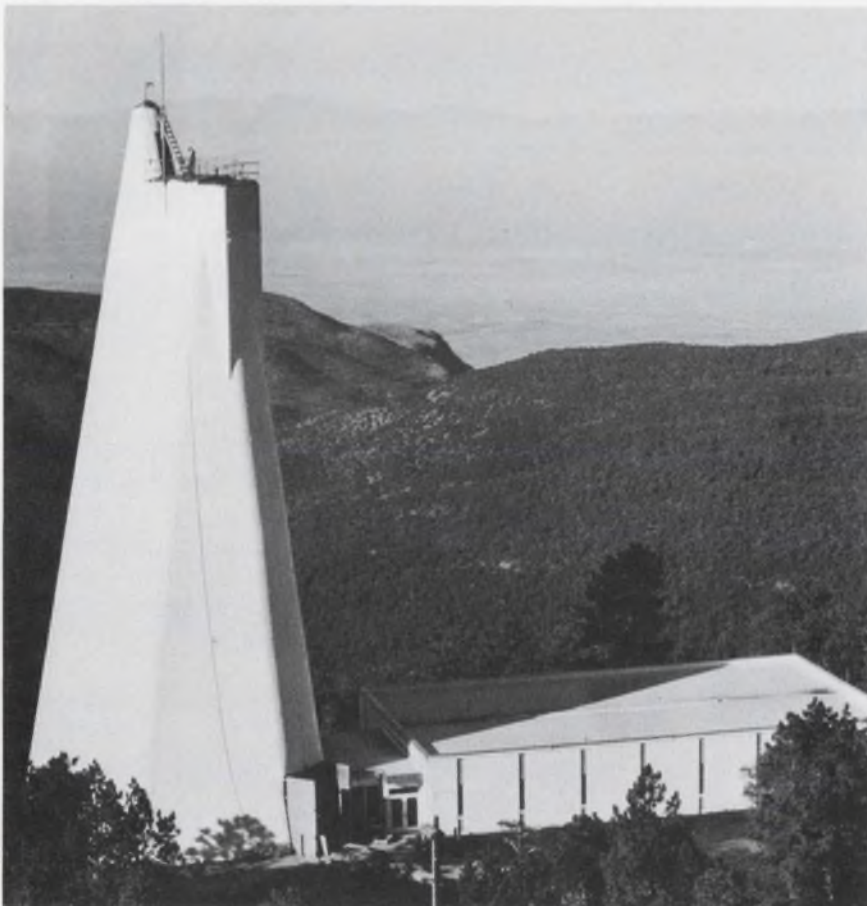
A 321-foot-long vacuum chamber will enable this solar telescope to provide high-resolution, jitter-free pictures of hitherto unseen solar activity.
