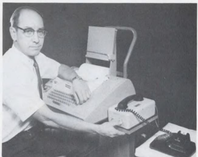
With the flip of a switch, author Roubique converts his teletypewriter into a time-shared terminal that operates over conventional telephone lines.
