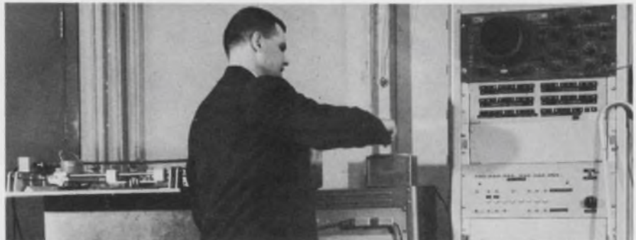
MIT reading machine for the blind has flying-spot scanner (left) that uses oscilloscope as light source. It reads type aloud, one letter at a time.
