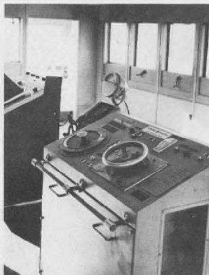
Bridge console in General Electric system allows complete control of the ship's propeller speed from "full ahead" to "full astern."
