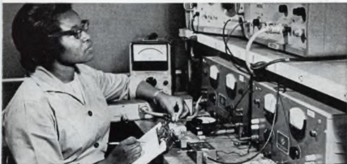
100% testing for 450 Mc/s gain and noise figure
