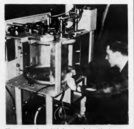
Klystron carrier, which is part of the Aleutian communications project, is unpacked and assembled by Western Electric engineer.
