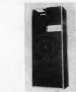
Complete rack consists of 4 independent modules holding five magazines of 20 transistors each, or 400 transistors per rack. Each module has two individual power supplies, a separate control circuit, interlock system and cycling instrumentation. Rack fits 44-1/2 x 78 x 32-1/2in. space.
