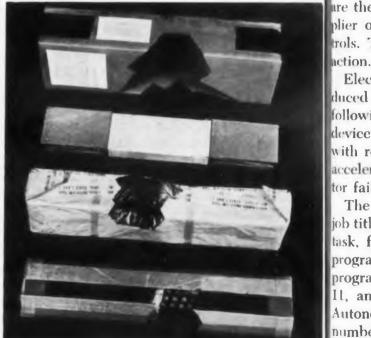
Packaging of component boards with parts soldered in place for shipment is illustrated. This interior package is wrapped in six sides with rubberized hair and entire packed in a larger exterior container.
