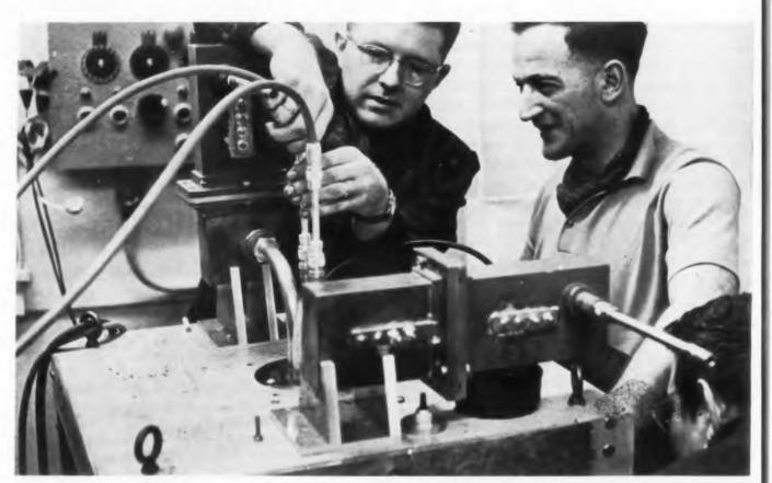
**Project Echo** receiver uses this maser, giving low noise reception considered virtually impossible to achieve a short five years ago. Other breakthroughs like this should permit much more efficient bandwidth utilization than can presently be foreseen.
