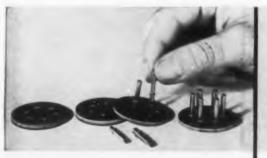
Vibration-free plug bases, fabricated by CDF. A special bond of CDF Dilecto laminated plastic and rubber.
