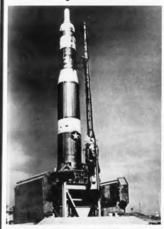
Titan ICBM check-out missile is in firing position in the underground launcher designed and built by American Machine & Foundry Co. of New York. The missile is fueled and guided from the underground launching complex. During the last few minutes of the ountdown the doors open and the missile raised to ground level for launching.
