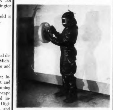
suit to protect against high-density rf radiation is nade of neoprene-coated nylon with nylon linings. Visor is wire mesh.
