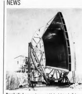
Parabolic horn antenna at Holmdel tracks Echo with minimum thermal noise. "There seems to be little room for improvement insofar as noise is concerned," said one Bell Labs engineer of the big horn. Maser amplifier and other receiving gear are housed in cab at the small end of the horn.
