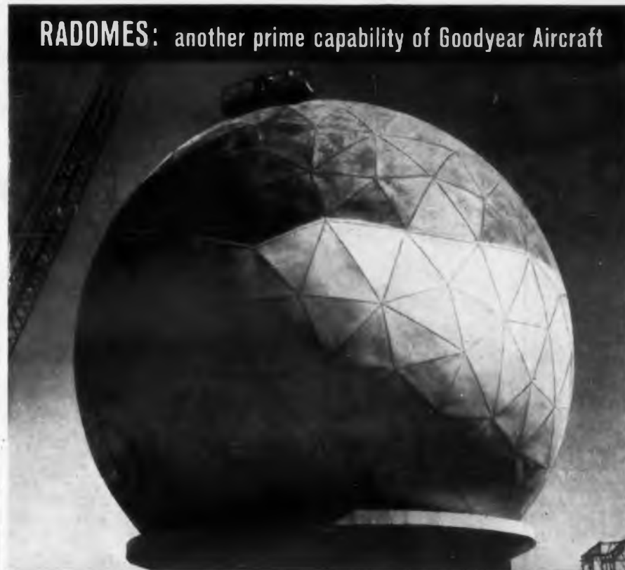
110-foot rigid radome, pioneered by GAC
