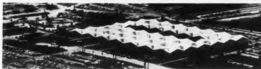
Currently doubling in size is the 310,000-sq ft TI Semiconductor-Components division plant, already the world's largest semiconductor facility.
