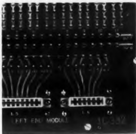
Fig. 2. Numbering system allows recording of temporary circuit for duplication later.
