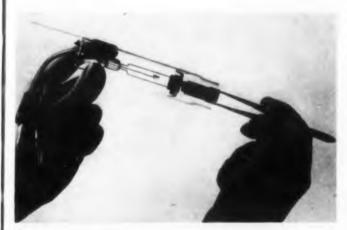
Experimental Westinghouse tube, with pinheadsize silicon-carbide crystal for emitter, could be forerunner of semiconductor electron tubes.
