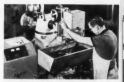
Metal disintegration, a fast, economical way Synthane uses to produce or revise dies.
