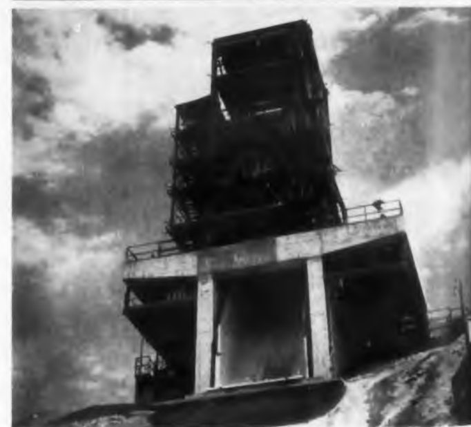
One of Lockheed's test stands with dynamic thrust mount to simulate flight environment.
