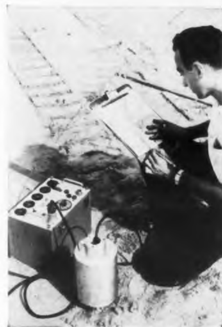
Nuclear-Chicago's new portable scaler uses five Sylvania counter tubes
