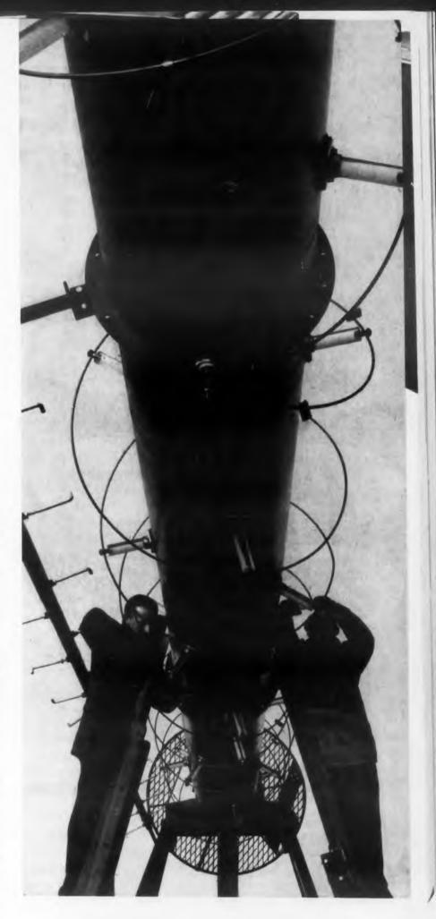
**TV Titan.**—This 57-feet-long, 5,500 pound helical television broadcast antenna will soon be blanketing the Seattle, Wash., area with VHF TV picture and sound signals. Designed by General Electric, Syracuse, N.Y., the antenna is self-deicing and can withstand severe lightning and other weather hazards.
