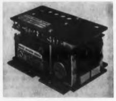
This line of static inverter supplies has been developed from similar items which the company has been building for some time. Covering a range of power ratings, the units are particularly suitable for gyro wheel supplies or where 400 cps accurate to  $\pm 0.01$  per cent is required. Waveform, simplicity of circuitry, fast starting time, and good voltage regulation are featured.
