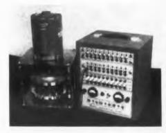
This read-write system for magnetic tape or drum memories measures 11 in. high x 11 in. wide x 9 in. deep. Individual units are entirely transistorized and printed
