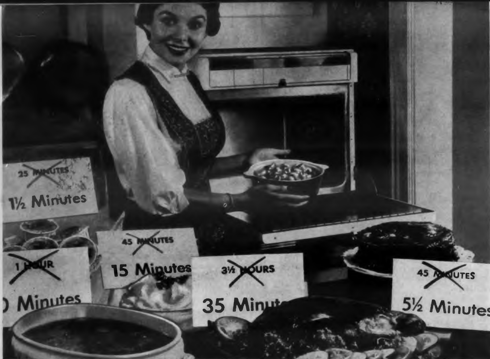
Microwave cooking shaves hours from food preparation time. This is a home-type electronic oven developed by Raytheon for production by appliance manufacturers.
