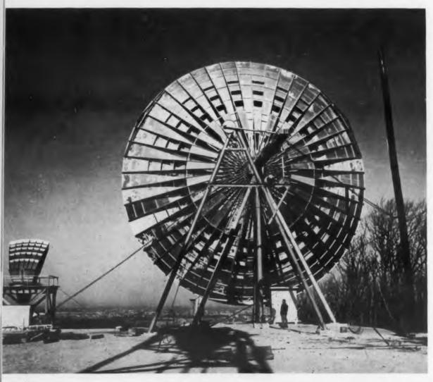
Over-the-horizon microwave transmission is accomplished with this 60' diameter experimental antenna. It has 30 times the surface area of the conventional antenna at left. The new method of transmission should be very valuable in overwater relaying or over rugged territory where it is difficult to establish the conventional type of radio relay system. The new method is expected to supplement than replace conventional equipment.
