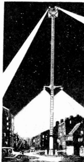
France Lights the Way to Better Traffic Direction The quaint little town of St. Denis, France, has recently inaugurated what is regarded as the tallest traffic tower in existence. Four searchlights, eighty feet above the ground, project in each direction. Half-way up the tower are brilliant lights which illuminate the square.
