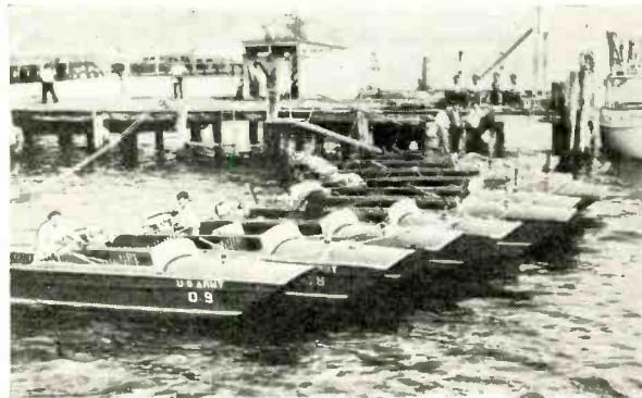
Courtesy Johnson Motor Co. A group of the U. S. Army Air Corps' speedy rescue boats, equipped with outboard motors and three-blade propellers. They are being utilized to lessen the hazards of emergency landings of planes.
