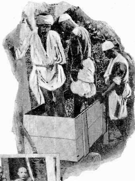
A three-man primitive pump for irrigating rice fields in South India. Two of the men walk back and forth on the suspended pole, balancing themselves with sticks.
