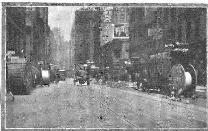
Photos New York Telephone Company
