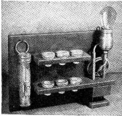
The fuse rack and test lamp outfit complete, with flashlight for emergency use.
