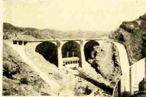
A view of the Coolidge Dam in Arizona showing spillways on either side of the power house.
