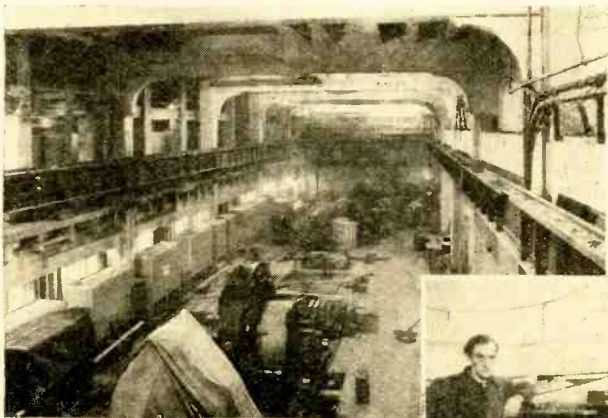
The two ton storage batteries seven feet long, two feet wide and two feet nine inches deep were placed on special wheeled trucks and hauled through an underground tunnel to the new location.
