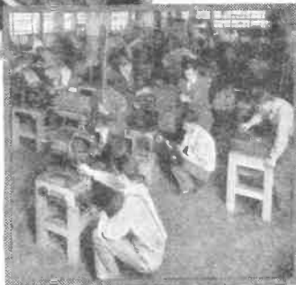
These Coyne men are connecting up, testing, and repairing A. C. motors and controls.
