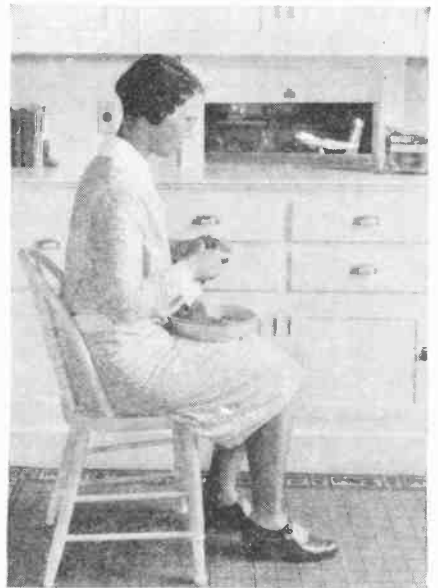
Transfer food through a two-way pass closet between kitchen and dining room.
