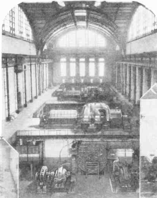
In the turbine hall of the Philadelphia Electric Company at Port Richmond, two steam turbo-generator units develop 120,000 k. w. At the left is pictured the turbine room of the company's Conowingo plant, costing $52,000,000, where seven 54,000-k.w. hydroelectric units supply the Philadelphia territory. Note size of workman.
