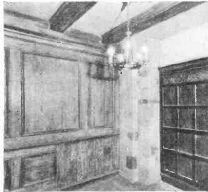
Paint on plaster here provides a striking imitation of wood and stone. (The Stone-tone Company.)
