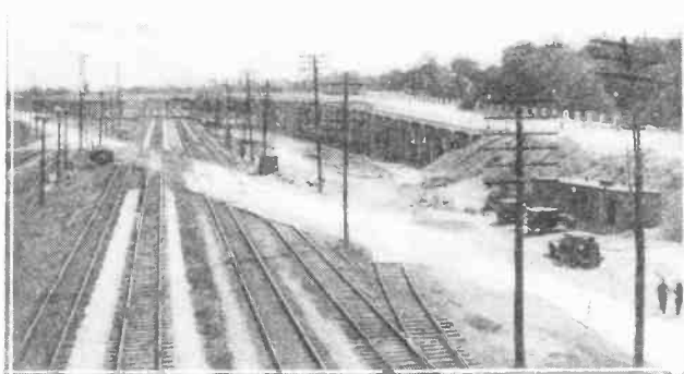
This bridge structure in the south end of Cleveland carries a highway safely across two steam and one electric interurban lines.
