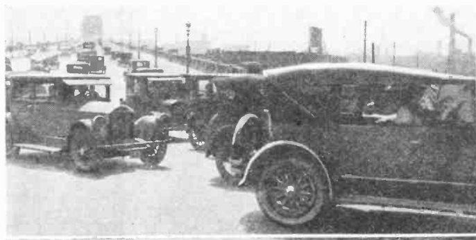
More than 64,000 vehicles have been counted in a single day using the western approach to Superior high-level bridge, which crosses the Cuyahoga Valley.
