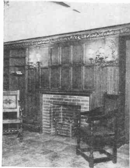
Wall panels of asbestos composition have an amazing resemblance to real oak. (Lyon and Taylor, Architects.)
