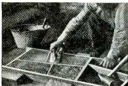
The trowel is worked along the sides of the forms to obtain a close contact.
