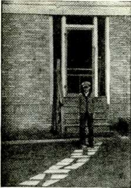
The above illustration shows the completed walk with blocks set in the ground, so that they will not interfere with the lawn mower.
