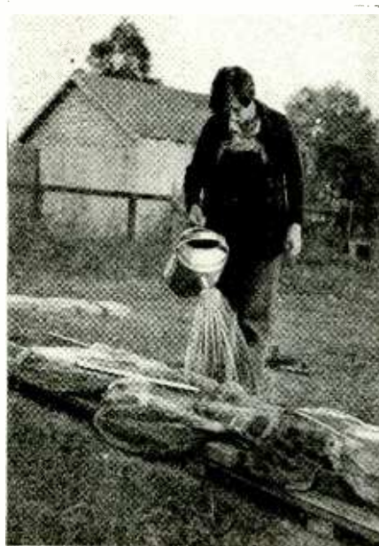
Covering the concrete and wetting the cover occasionally results in a stronger product.
