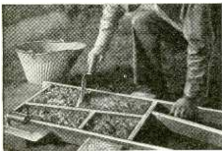
The upper surface of the concrete is worked with a trowel until it becomes smooth.
