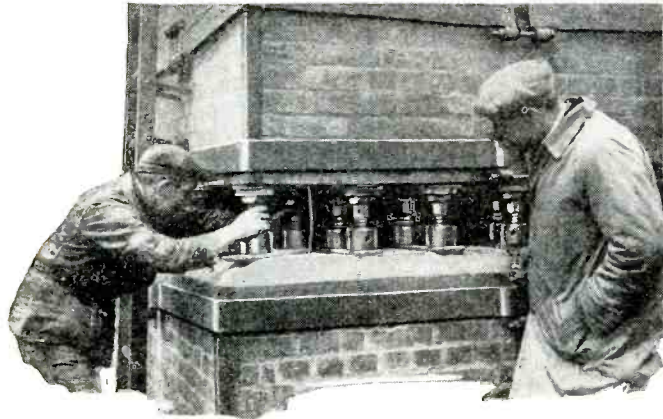
Photographs above show a surgical operation on a chimney. The chimney leaned as is indicated in the photo at the right. After being girdled with straps, some of the bricks were removed, and jacks inserted. These were lowered a thousandth of an inch at a time, and the chimney straightened.
