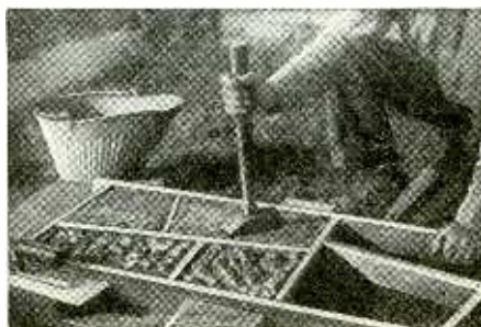
Thorough packing of the mortar in the forms is important. This process is illustrated in the above photograph.
