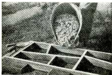
A coal scuttle is excellent for pouring the mixture. Note stiffness of mortar.
