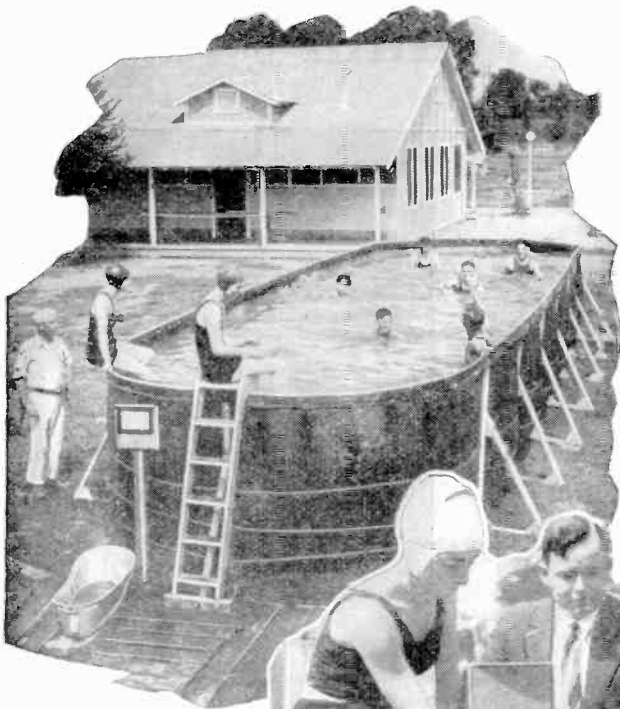
Tourists arriving in Washington, D. C., find a huge portable swimming pool at their disposal. The pool is 40 ft. long, 10 ft. wide, and 4 ft. 9 inches deep. As may be seen in the above photo, it is constructed entirely of waterproof canvas supported by a steel framework. The pool is readily portable, and can be set up in two hours' time. Several ladders placed around the edge provide entrance and exit to and from the pool.
