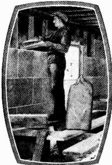
Above—dry insulation being poured behind the gypsum wall board.
