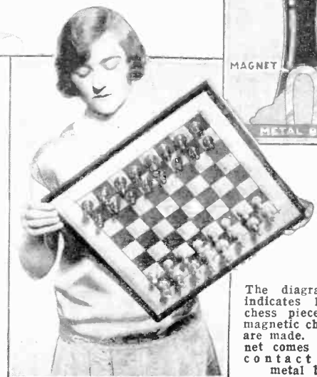
MAGNETIC CHESS BOARD —The playing pieces of this chess board are magnetized so as to hold the set to the metal board, regardless of the position of the board.
