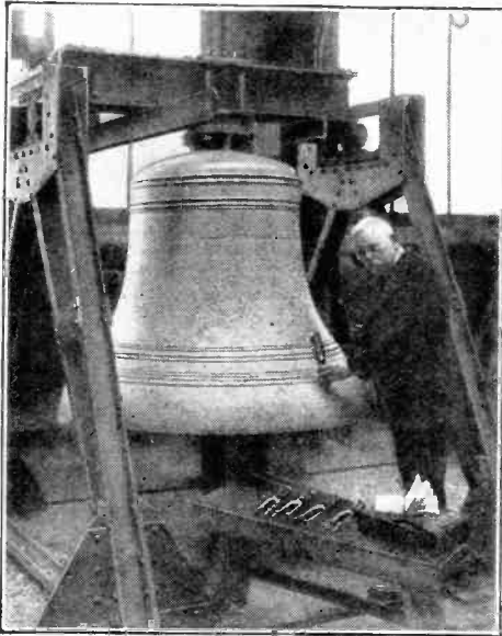
Tuning forks are sometimes used in tuning bells, but when groups of bells are made, the experienced ears of the bell makers are usually relied on.
